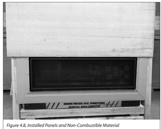
Figure 4.8, Installed Panels and Non-Combustible Material
